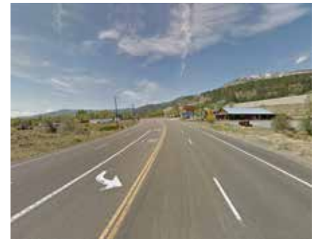
Existing condition through Old Washoe City.
